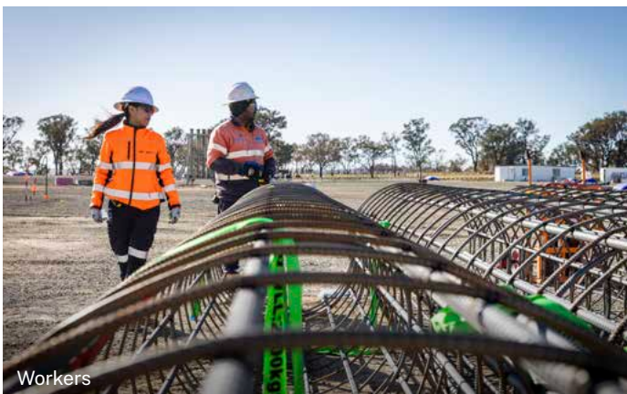
Tower construction underway
