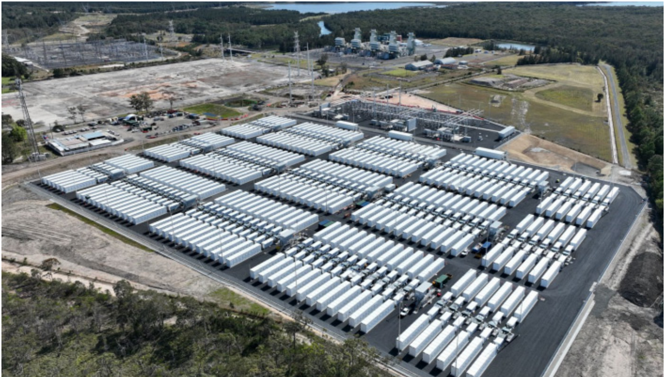
Figure 5: Construction of the Waratah Super Battery at the Lake Munmorah site
