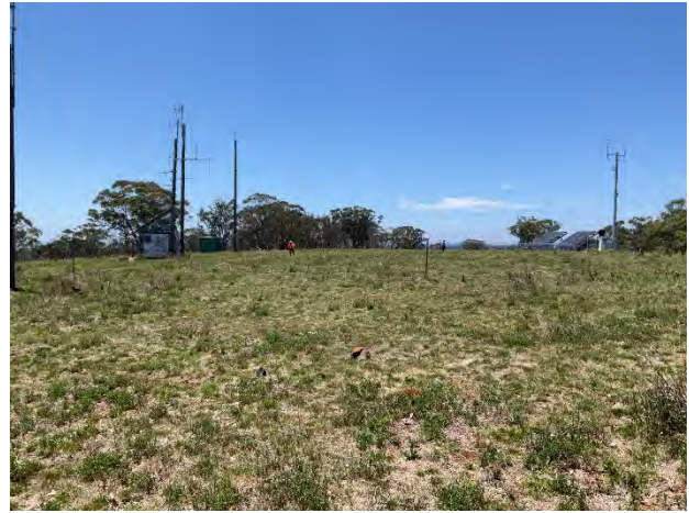
Plate 4.16 Communication infrastructure on the gently undulating flats in SU 16, facing north
