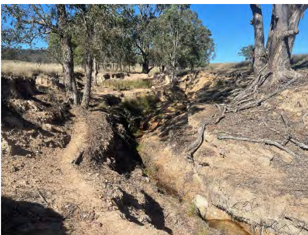
Plate 4.57 Excavations at Whites Creek, facing north-west
