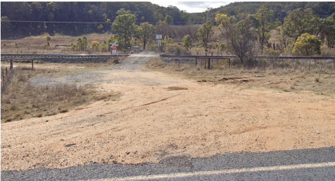
Figure 3-10 Existing passive control rail crossing (Google Street View, August 2023)
