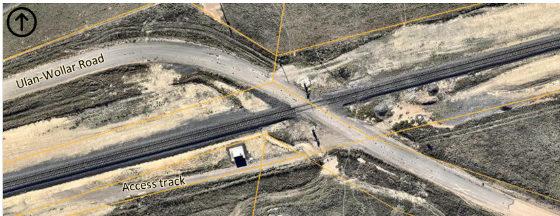
Figure 3-14 Existing access track intersection with Ulan-Wollar Road (Nearmap, May 2015)
