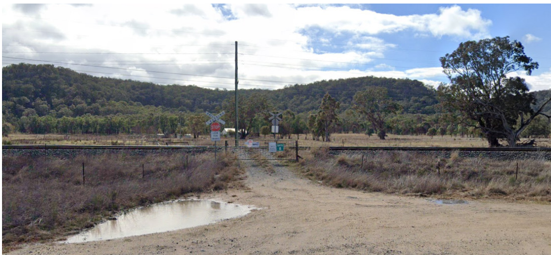
Figure 3-18 Existing passive control rail crossing (Google Street View, August 2023)
