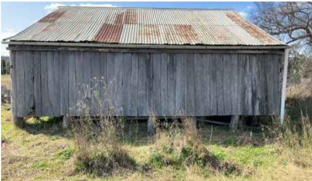
Plate A.108 Shearing shed southern wall
