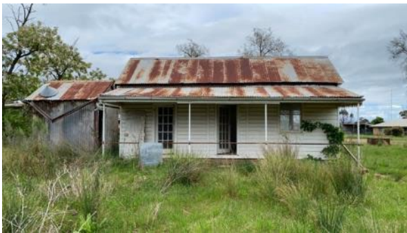
Plate A.3 Structure #1 looking west
