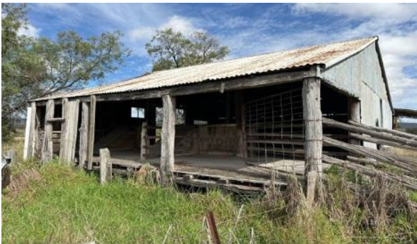
Plate A.110 Shearing shed northern wall
