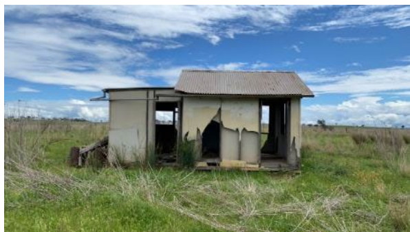
Plate A.19 Structure #10 looking west
