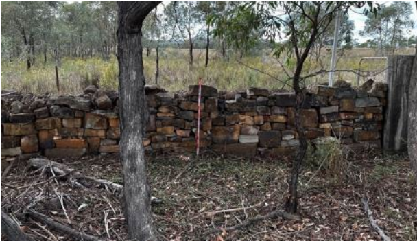
Plate A.106 Dry stone wall at entrance
