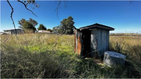
Plate A.54 Outhouse looking north-east
