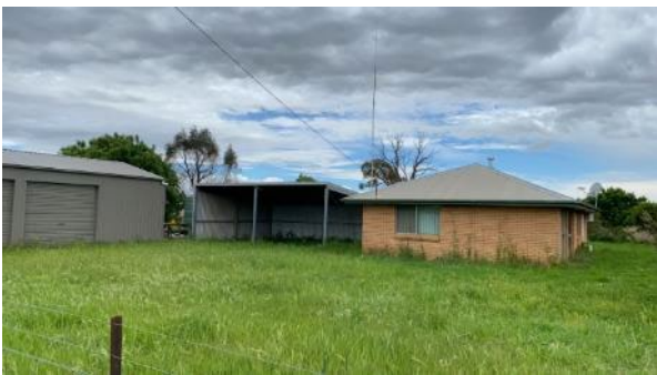
Plate A.14 Structure #8 looking south
