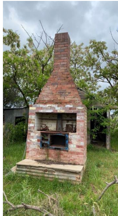
Plate A.12 Structure #7 looking south
