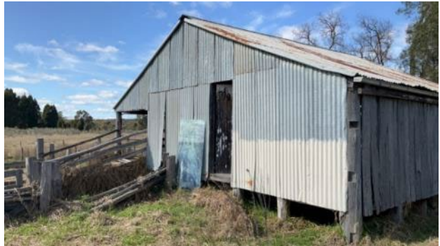
Plate A.109 Shearing shed western wall
