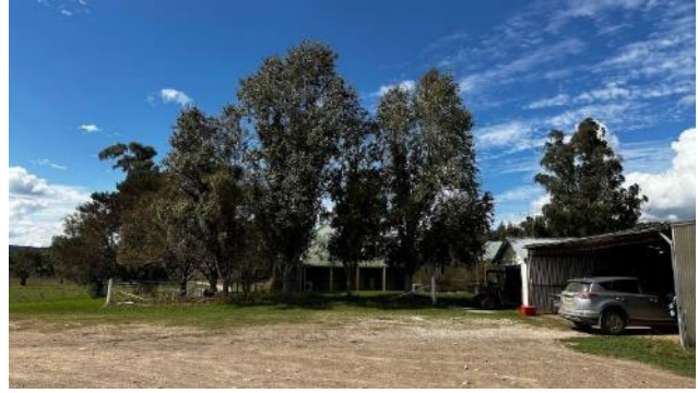
Plate A.123 The rear of Wandoona Homestead looking east
