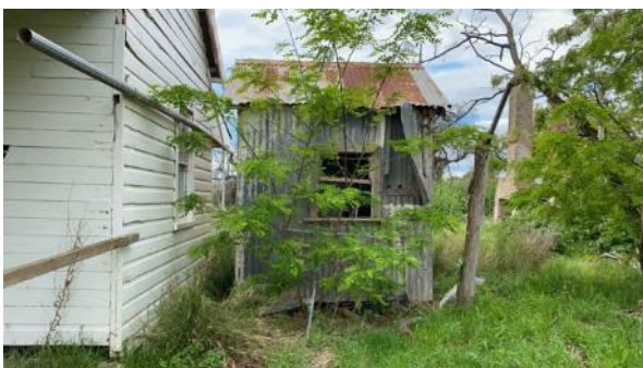
Plate A.5 Structure #2 looking east
