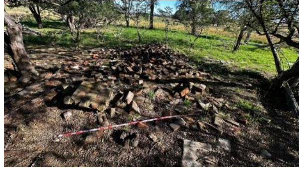
Plate A.82 Collapsed chimney
