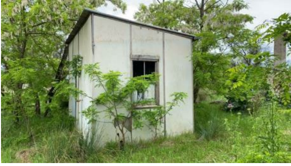
Plate A.7 Structure #3 looking north
