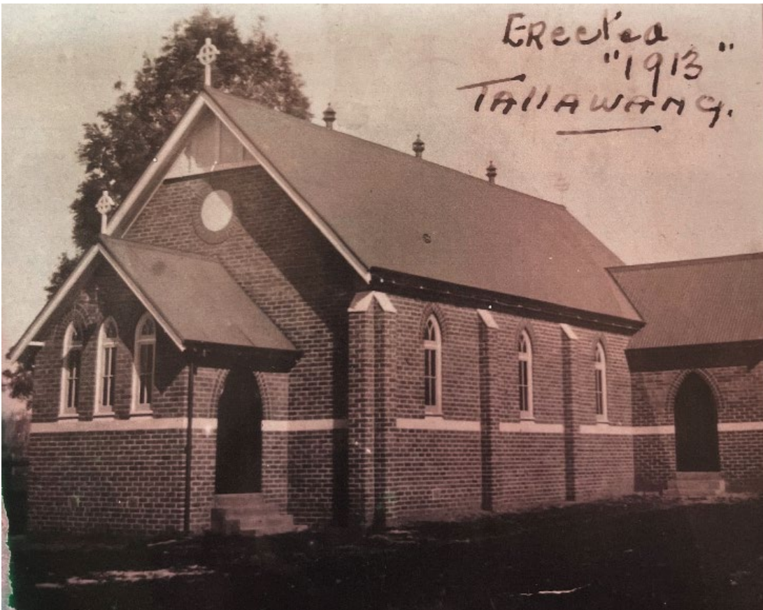
Plate A.72 St Paul's Catholic Church erected in 1913
