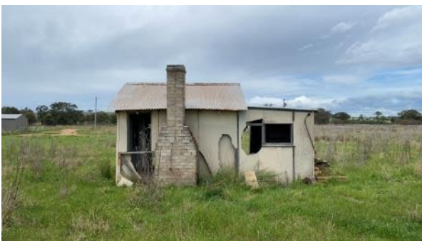
Plate A.18 Structure #10 looking east
