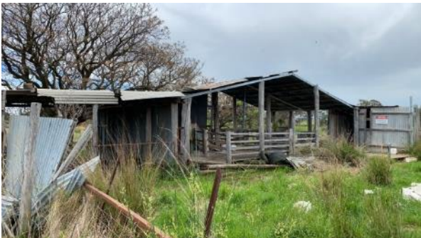
Plate A.16 Shearing shed
