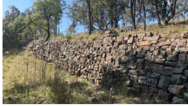
Plate A.104 Context shot showing embankment and stone wall
