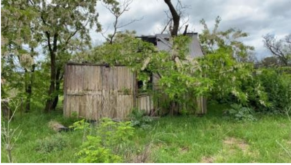
Plate A.9 Structure #4 looking south
