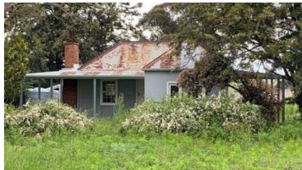
Plate A.49 Cottage looking south
