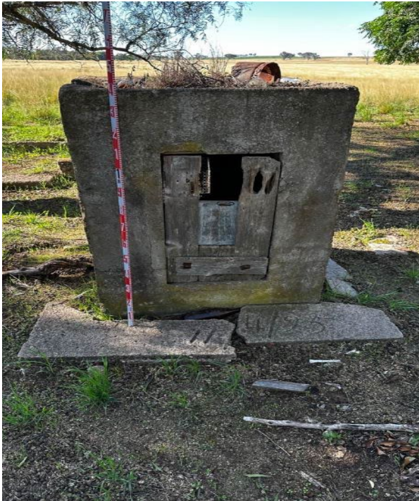
Plate A.83 Concrete meat safe with timber door and ornate metal grill dated to 11/4/1925
