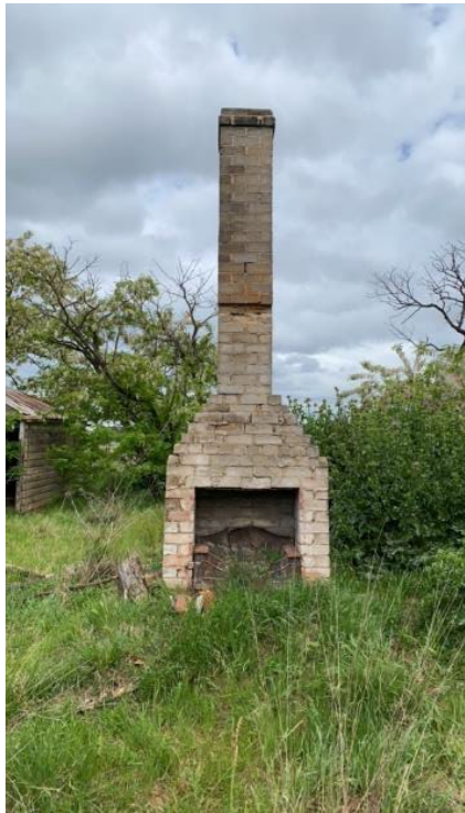
Plate A.11 Structure #6 looking south
