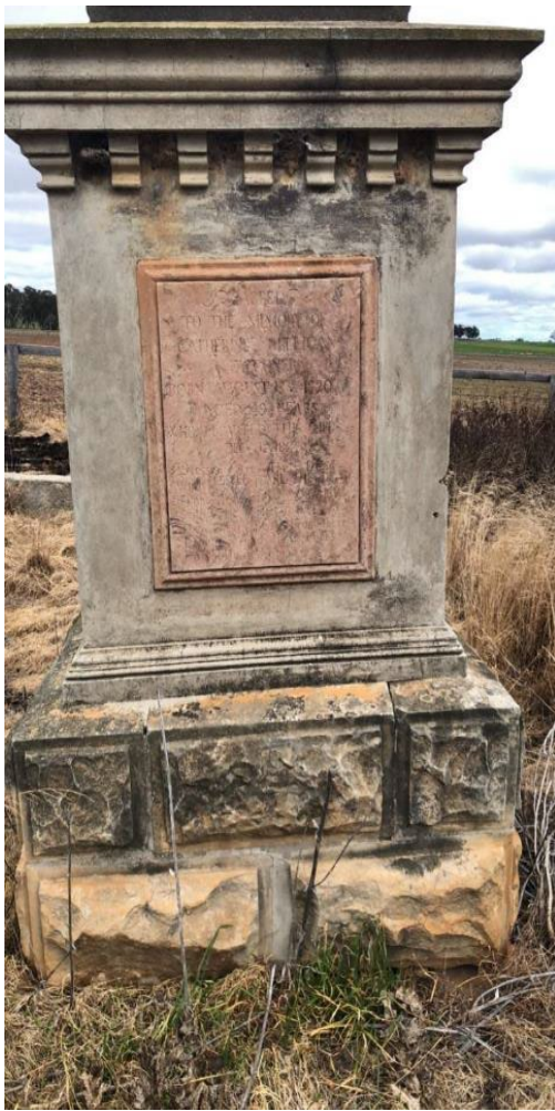
Plate A.41 Detail shot of obelisk plaque, note the angle of lean
