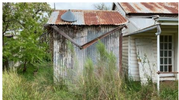
Plate A.6 Structure #2 looking west
