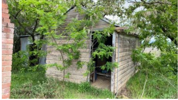
Plate A.10 Structure #5 looking south
