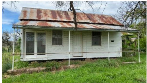
Plate A.4 Structure #1 looking east
