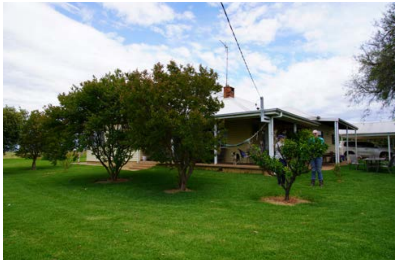
Photo showing dwelling aspect
