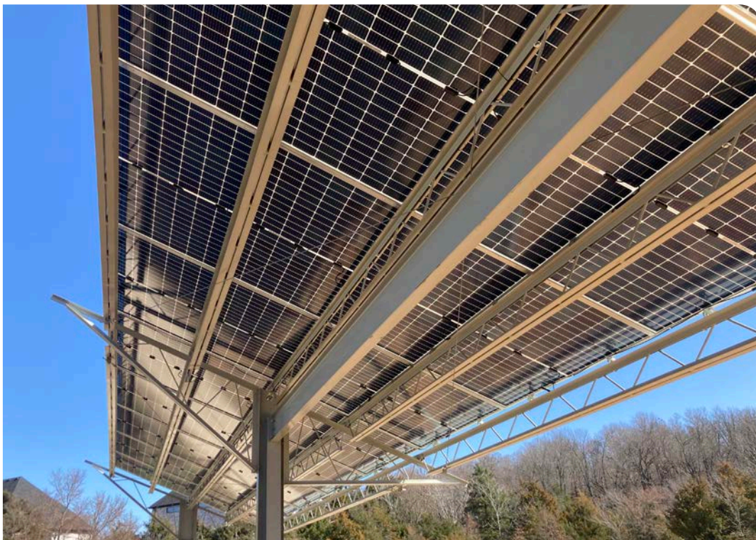
Photo courtesy of AgRack – MAS – bifacial solar panels
