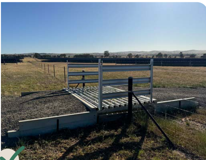
Retrofitted internal fencing and access grid
